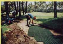
3 Lay Grass-Cel Turf Paving Blocks into prepared area.
