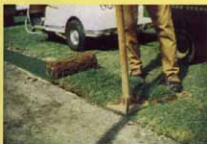
4 Replace grass over the top of Grass-Cel Turf Paving Blocks and tamp or roll in position.
