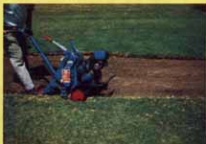
1 Cut grass from area to be laid with Grass-Cel Turf Paving Blocks.
